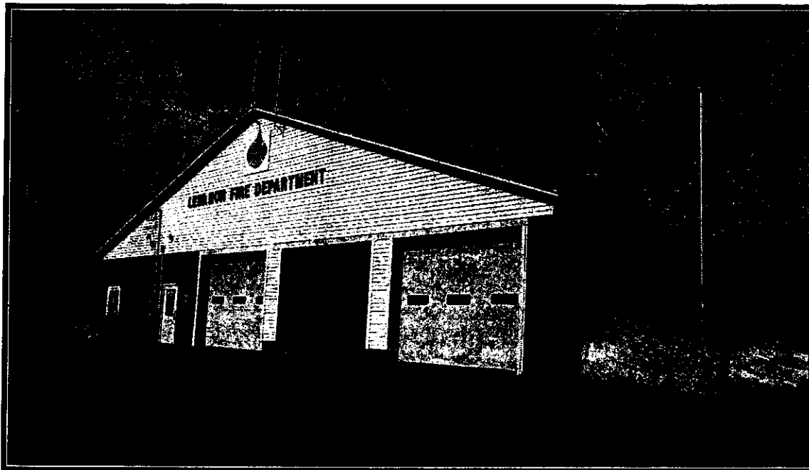
Photo 7: 113 Depot Road – Front of building.
