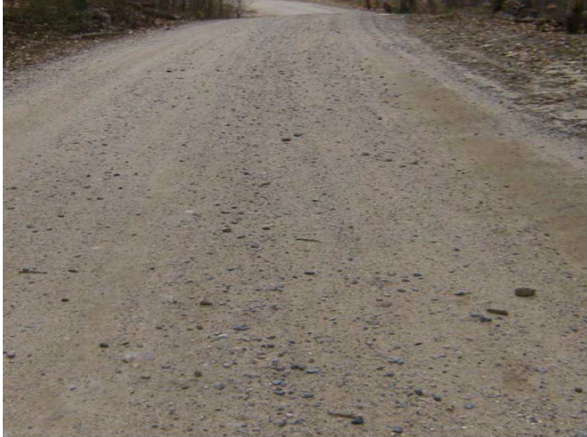
Loose Aggregate - Maine Local Roads Center Image
