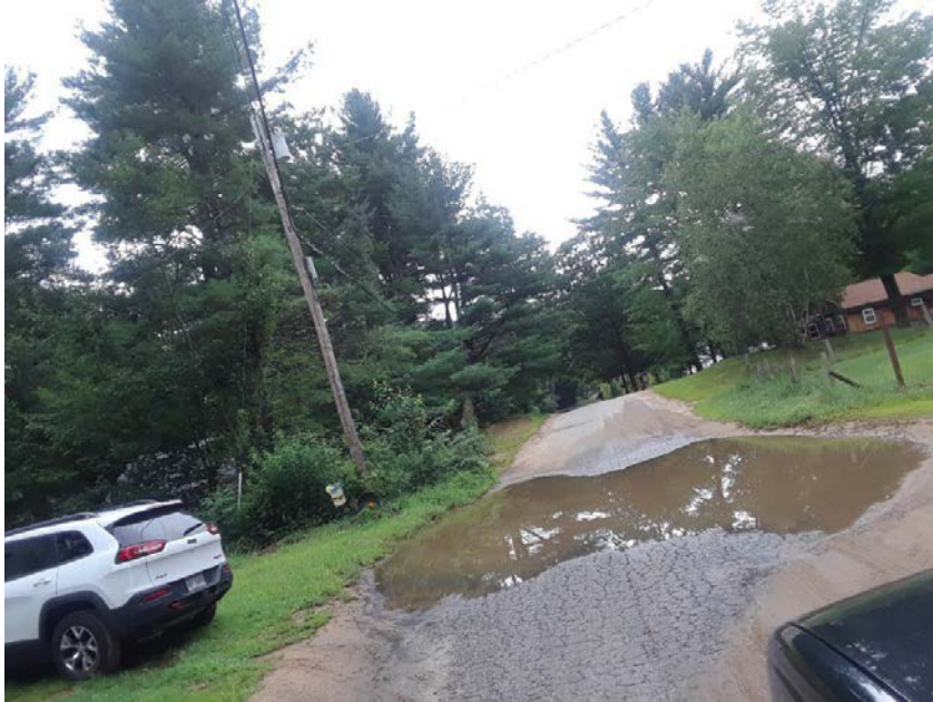
Roadside Drainage - Indian Lake Drive
