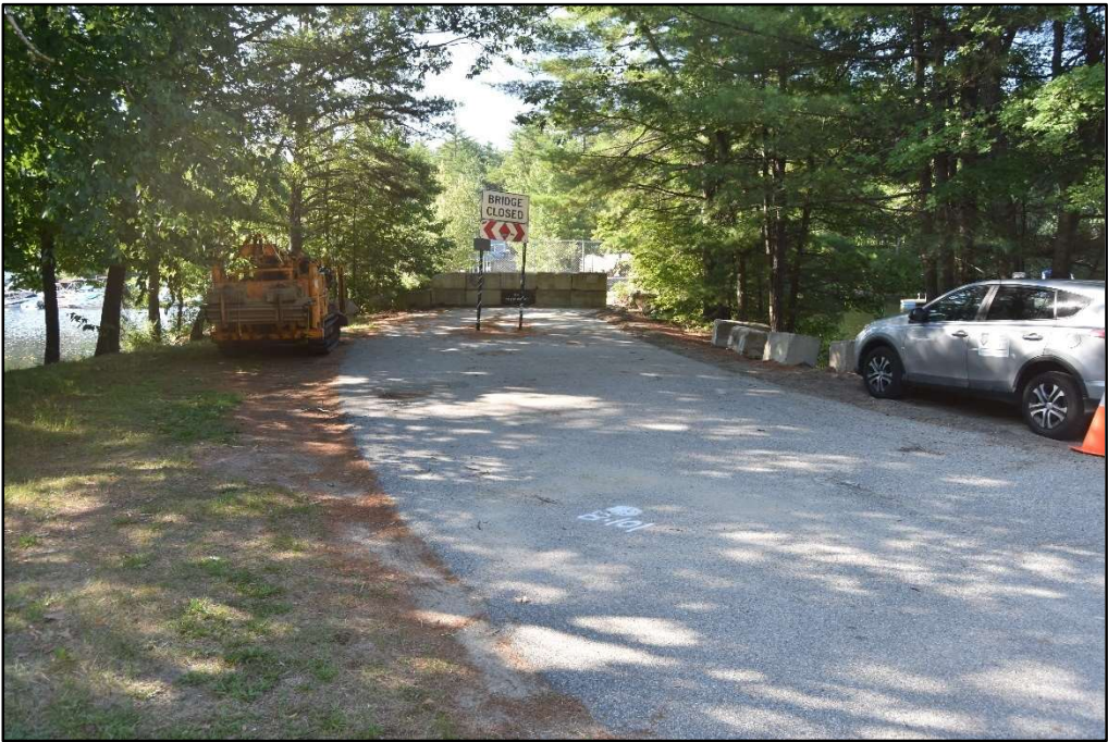
Figure 8. Conditions around the bridge location in Milton, view south.
