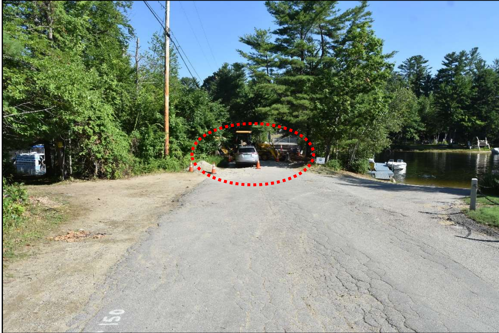
Figure 13. General conditions around the bridge (circled) in Lebanon, view north-northwest.
