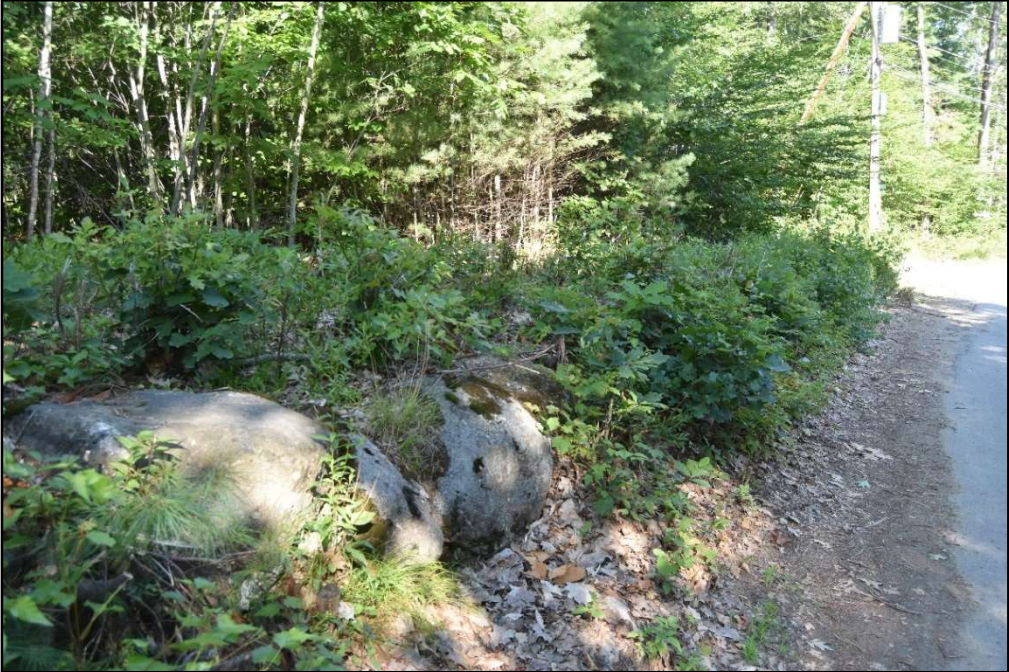
Figure 15. Cut bank along the western road edge, view northwest.
